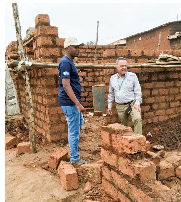
RedR's Val Tarasov supervises the construction of WASH facilities in a refugee camp in Rwanda.
