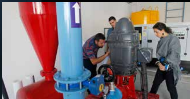
Danielle and colleagues check the flow meter and pressure gauge on a new water pump.
